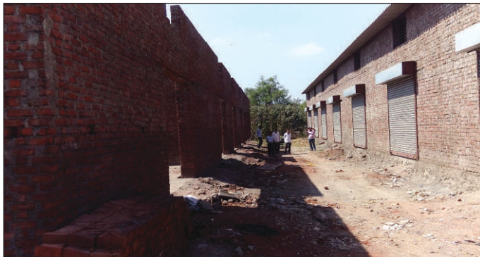
Infrastructure Development work is in progress like water connection, electricity connection and all in kharegoan, Thane
